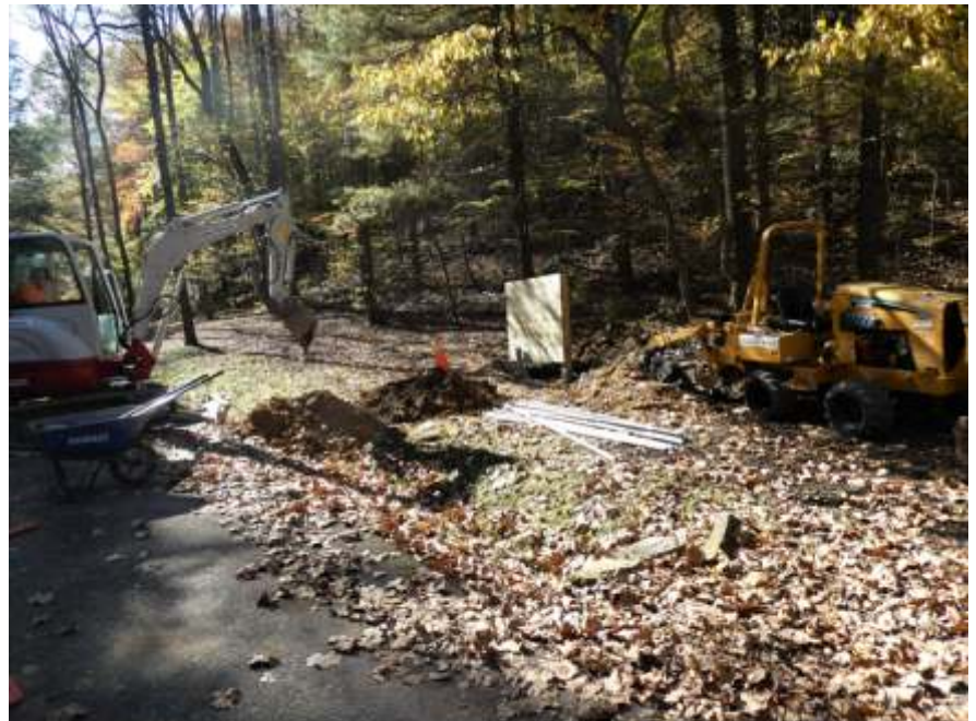
Electrical work in the campground.
