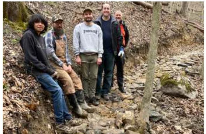
KVTA team pave a section of Middle Ridge Trail.
