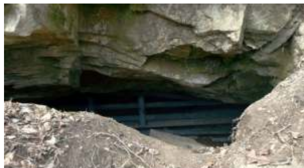
Installed bat gate. D. Porter photo
