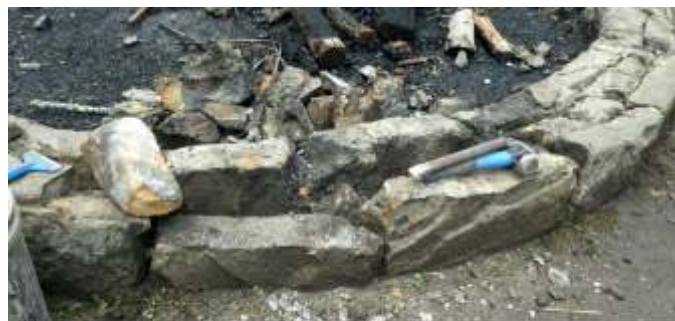
Removing the old cap with chisel and hammer.
