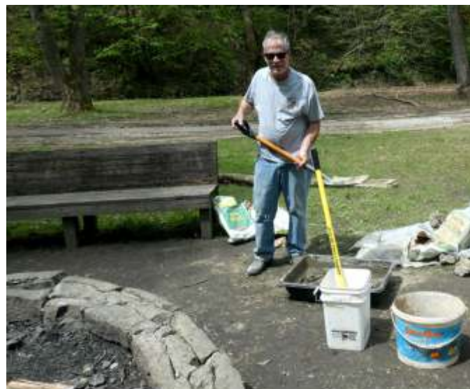
Foundation chairperson John Hughes mixing concrete.
